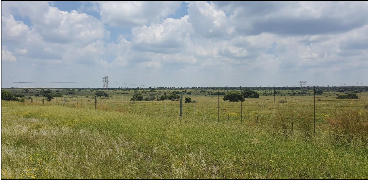
Figure 3-4: View of the project area
