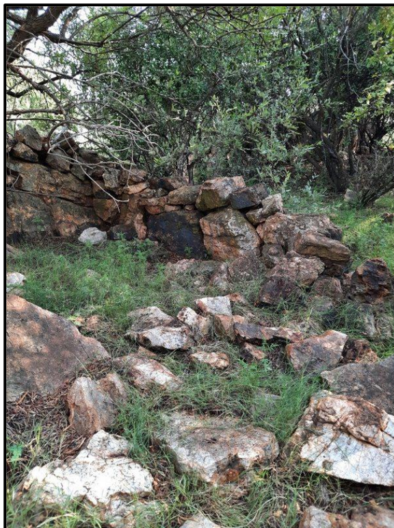
Stone packed enclosure at SF009
