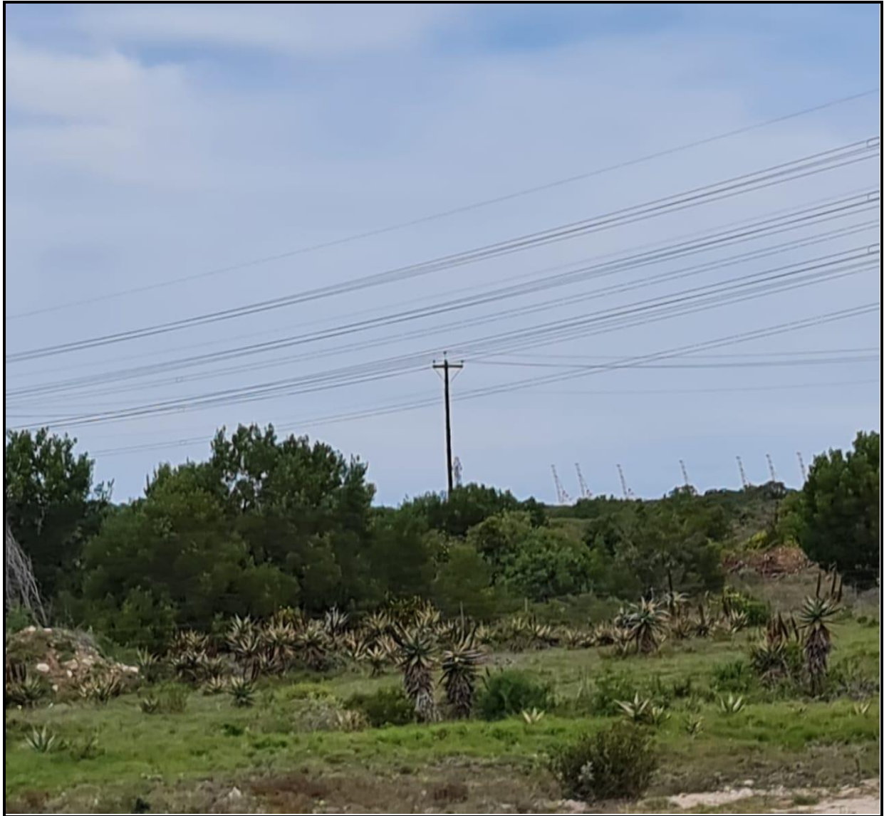
Figure 2: Existing 400kV powerline within the proposed location (Zone 7, 8 and 10) (Nsovo Site visit, 2020)
