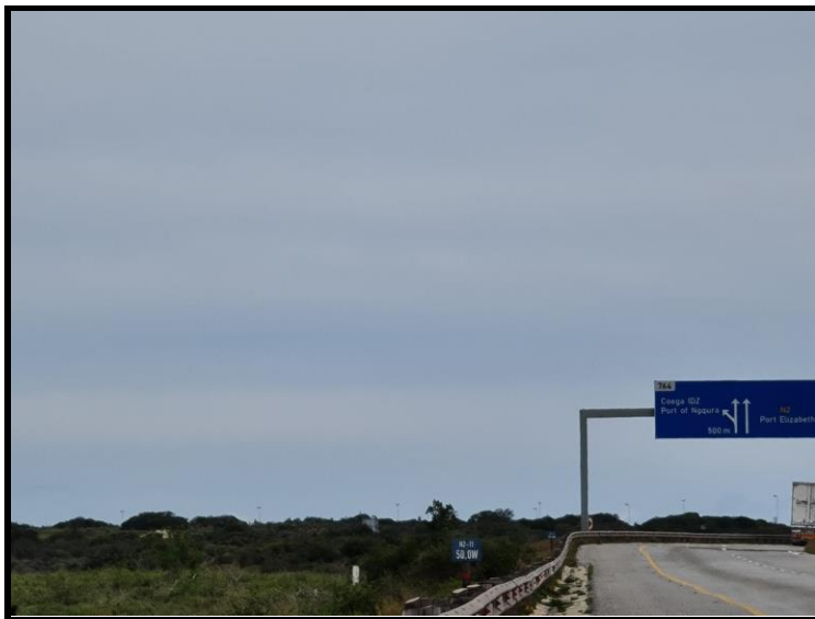
Figure 5: Access road (N2) to the Coega Special Economic Zone (SEZ) (site visit, 2020)
