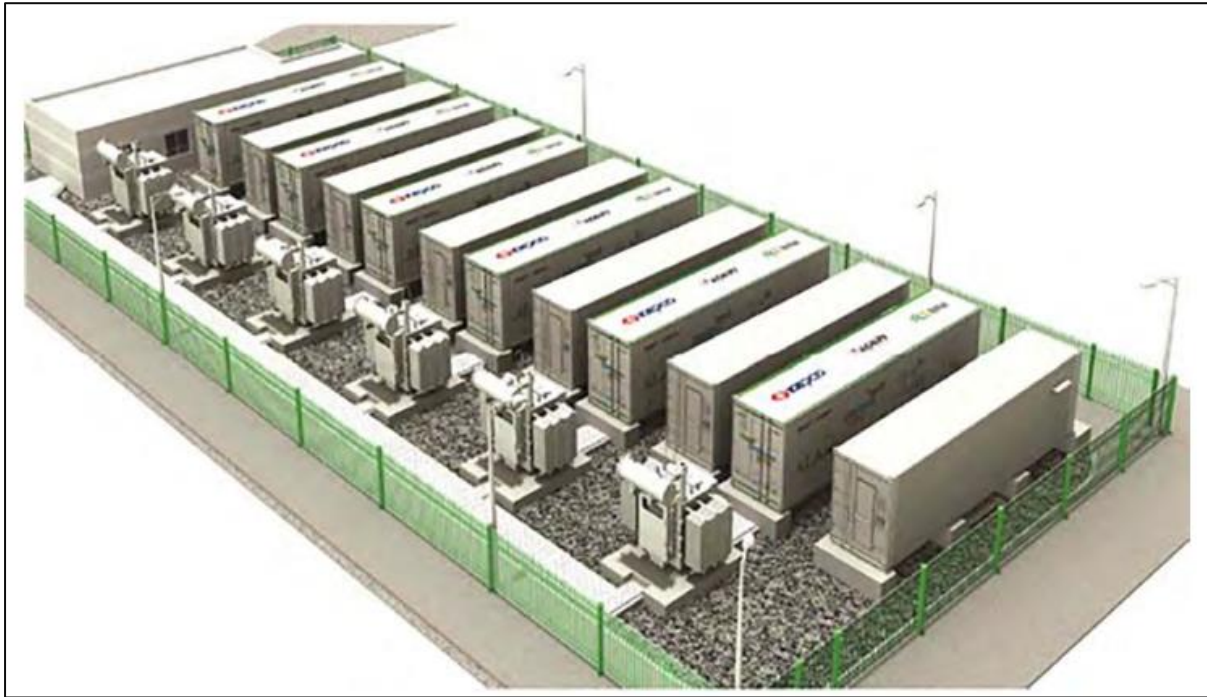
Figure 16: Graphic presentation of a Battery Energy Storage System (BESS).
