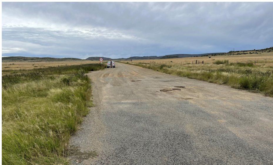
Figure 2.9: Potential Access Route Option 1: Divisional Road 3093 (Photograph taken from the R48) (Sturgeon, 2022)
