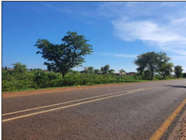
Figure 3-13: View of the alignment of Deviation 3 along the R524 road.
