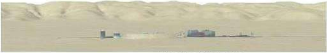
View from 5 000 metres
