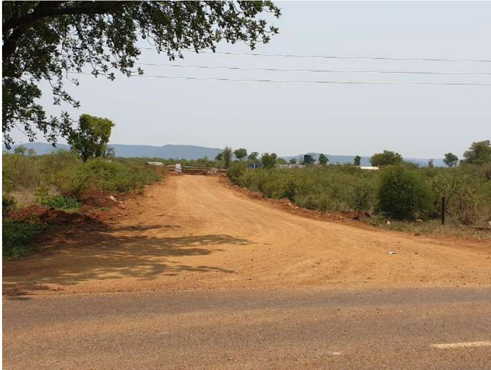
Photo 5: Deviation 3 facing West, the construction vehicles are busy constructing the Pennigotcha and Mhingaville substation located along Punda Maria road R524.
