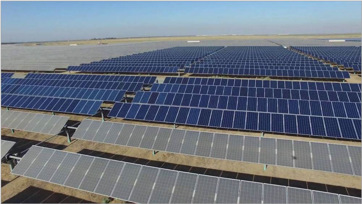
Figure 15: Example of Roads Between Trackers and Medium Voltage Substations (source: https://ecoinventos.com/ )
