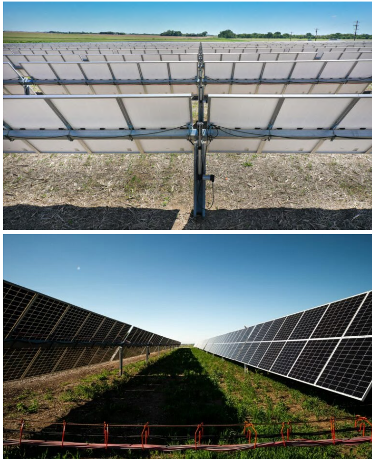
Figure 21: Monofacial (top) and bifacial (bottom) solar panels
