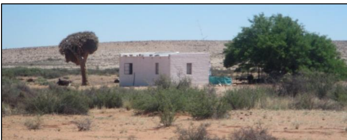
Figure 13: Farm houses on Pofadder 1 site
