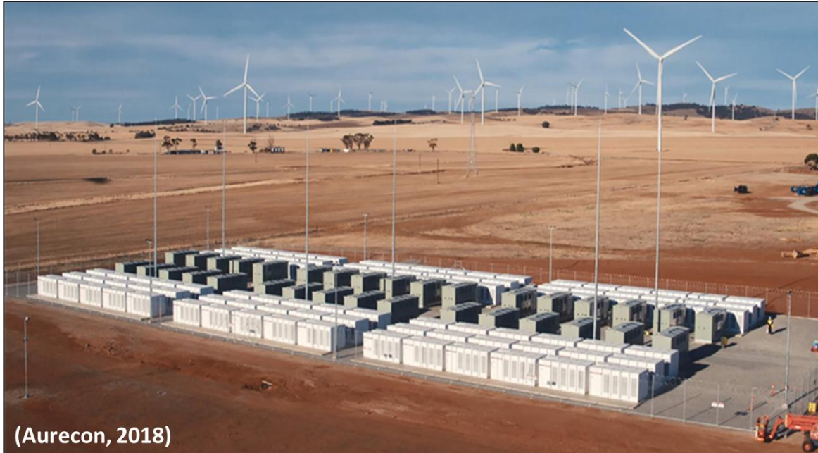
Figure 6: Example of a 100MW/129MWh Lithium-ion battery on the Hornsdale wind farm in Australia.
