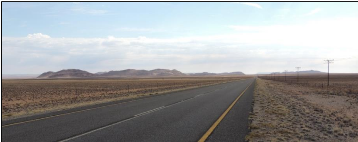
Figure 14: N14 National Road northbound just before Aggeneys Town
