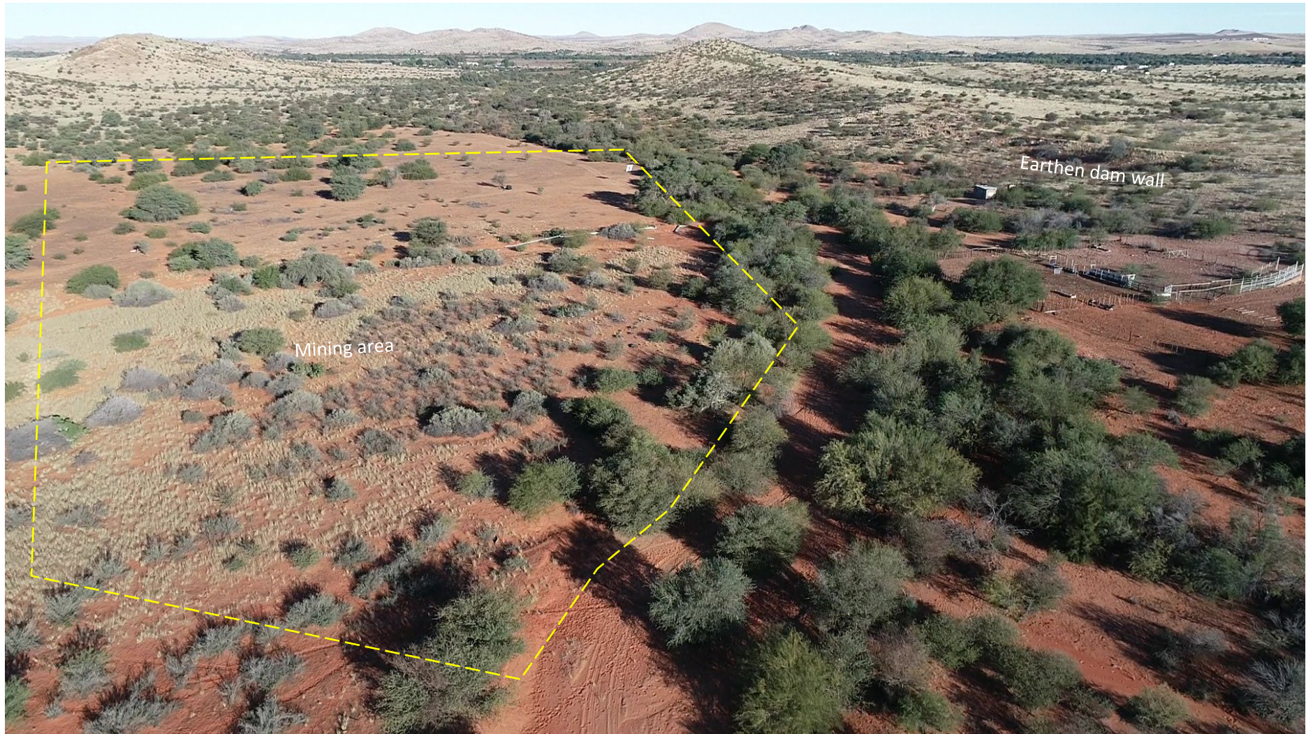
Photo 2: Mining area with sparse vegetation and showing remnant of historic irrigation plots. Also note earthen dam wall incorrectly identified as a wetland
