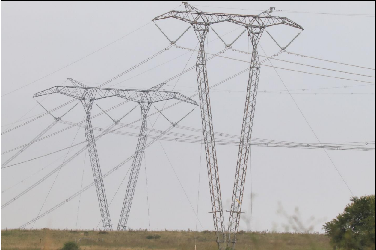
Figure 3. Photograph of the assessment area taken during field surveys.
