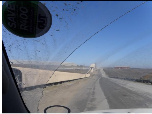
Existing overland conveyor from the power station to the radial stacker
