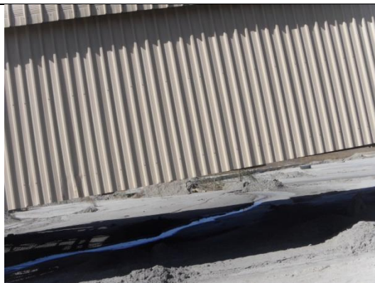
The section of the site underneath the conveyor system
