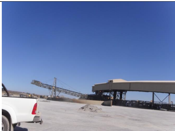
Existing radial stacker on flat terrain
