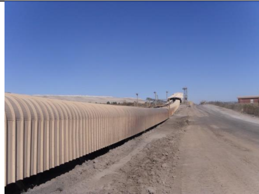
Flat terrain of the existing conveyor system
