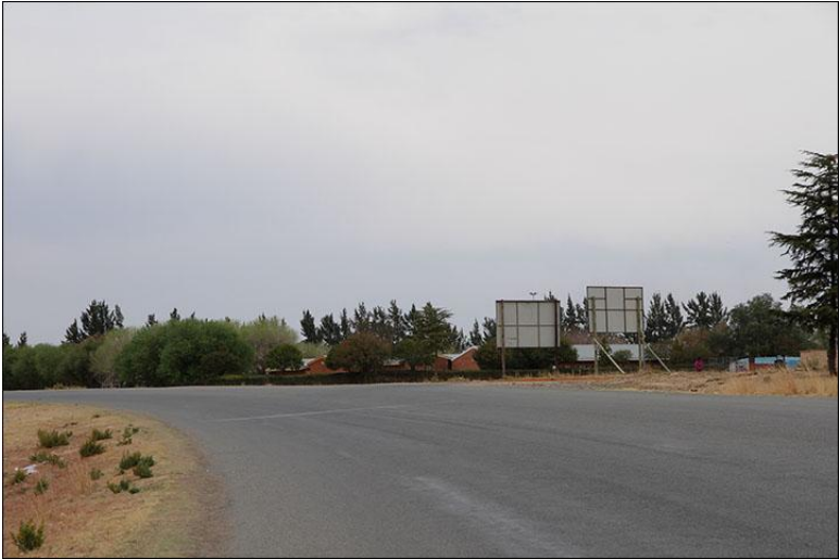
Photo 8: Intersection E as seen from the north
