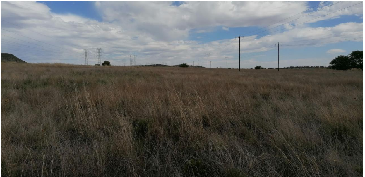
Figure 10: General view of part of the grid-connection site, looking south from the Harvard substation towards the site. The existing overhead lines can be seen to the left of the image.
