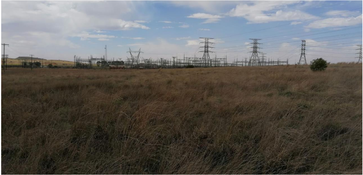
Figure 9: General view of part of the grid-connection site, looking north towards the Harvard substation.
