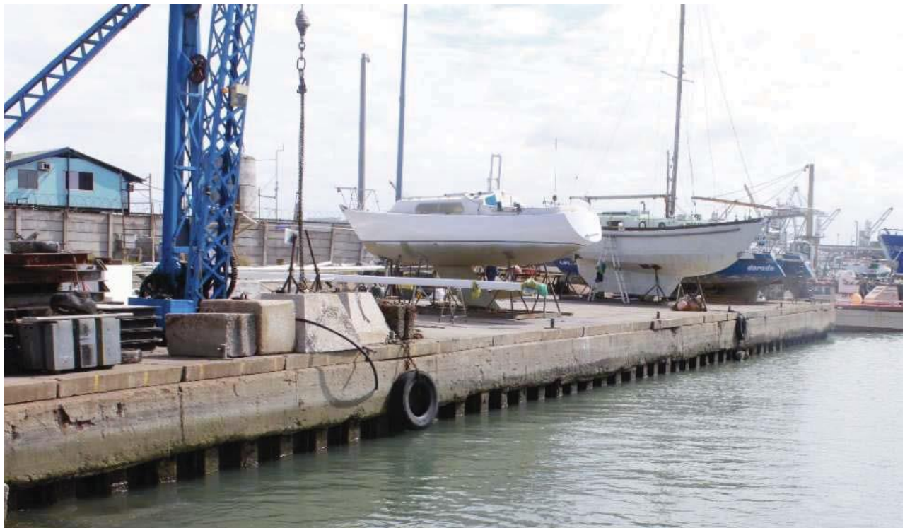
Figure 18: Southern side of the Old Tug Jetty sheet pile wall
