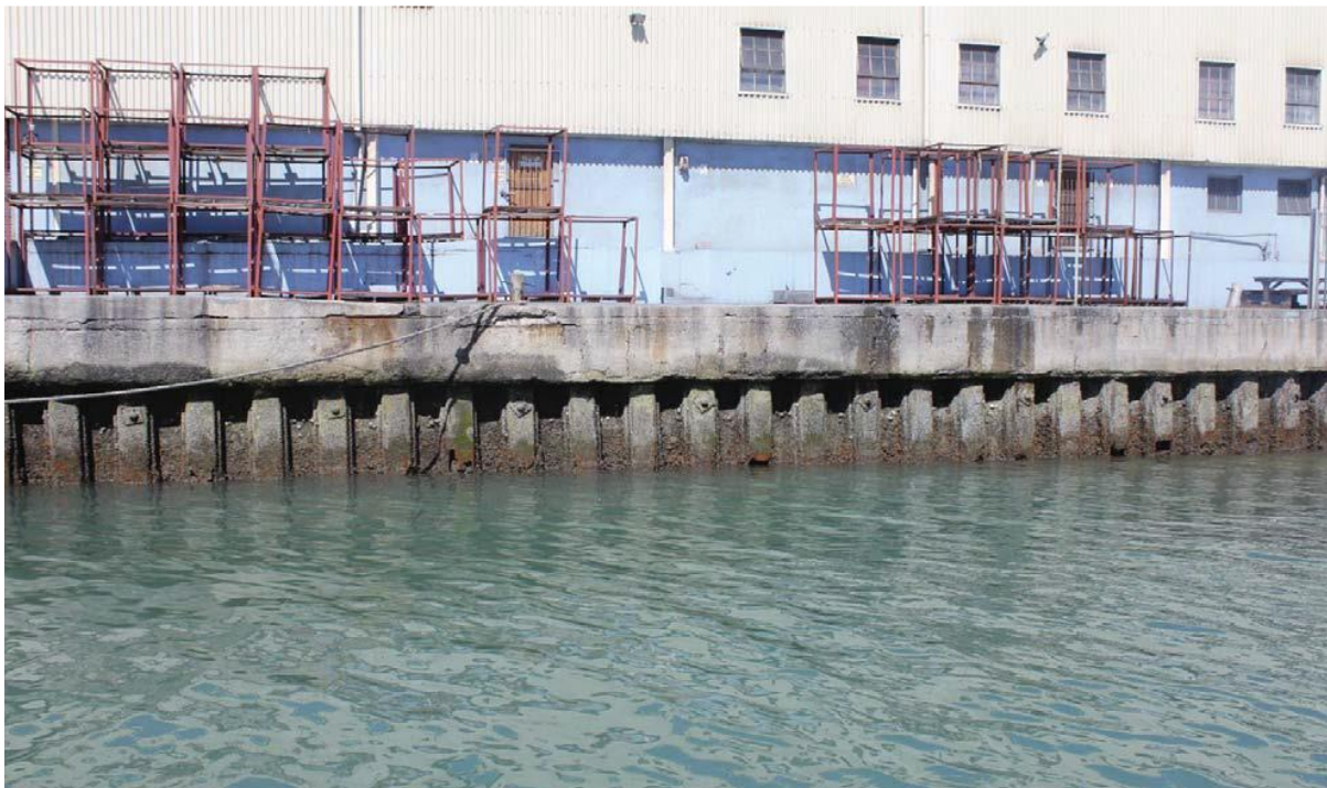
Figure 16: Old Tug Jetty Sheet Pile Wall
