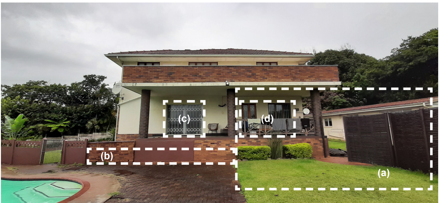
View 12: View looking at the north facade.
