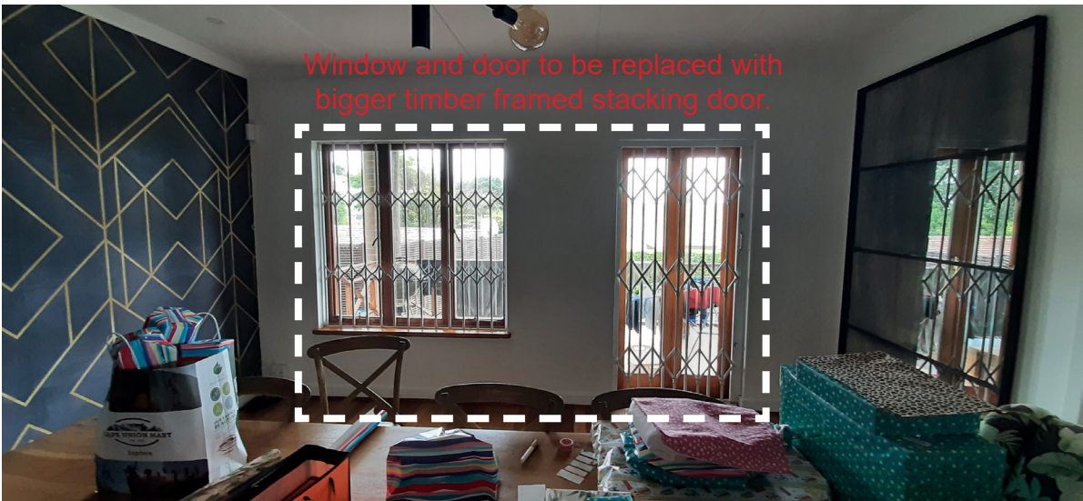
View 23: Internal view of existing dining room viewing northwards. Window and door to be removed and replaced with a timber stacking door (DF01-T02) for better connection to the new pavilion and pool area.
