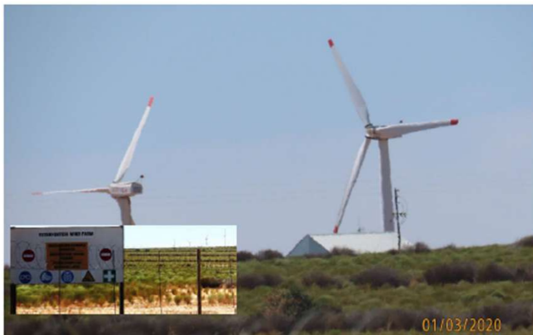
Figure 2: Red-tipped turbine-blades on turbines at the Ysterfontein wind farm north west of Clanwilliam in the Western Cape (S 32° 9'23.42" E 18°49'7.10"). While these mitigations are not used in the correct single-blade configuration used by the Norwegians, they set a precedent for turbine blades to be red-painted in South Africa © RE Simmons
