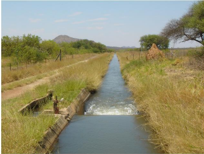
Photo 4: Main canal close to overflowing
