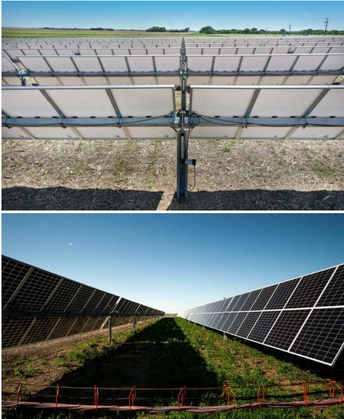
Figure 20: Monofacial (top) and bifacial (bottom) solar panels
