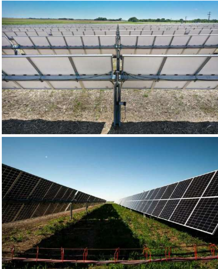
Figure 22: Monofacial (top) and bifacial (bottom) solar panels ( https://www.bluestemenergysolutions.com/bifacial-versus-monofacial-solar-panels-an-analysis/ )
