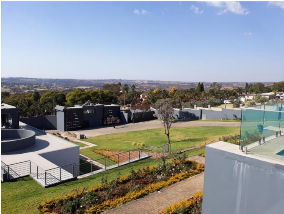
Figure 7: General view of the site.
