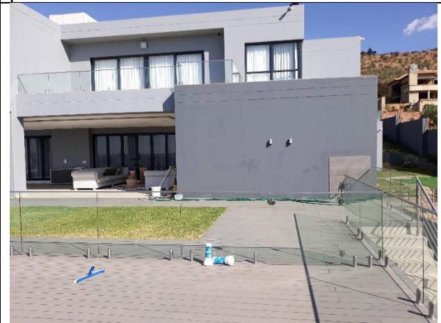
Photo 5: South west looking towards the main house.
