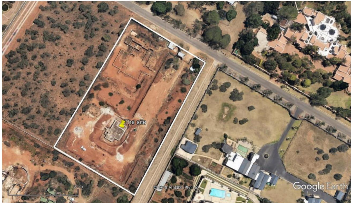
Figure 3: Detailed view of the site during construction.
