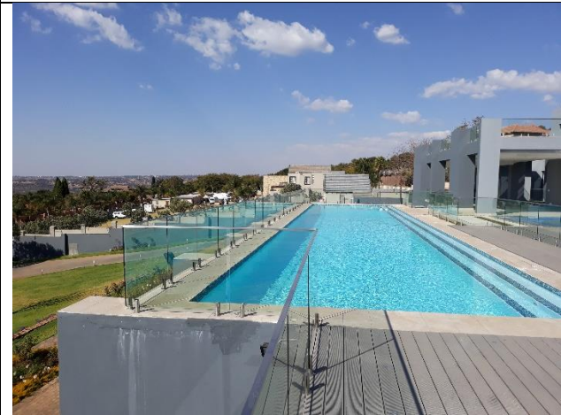
Photo 3: South east looking over the swimming pool.
