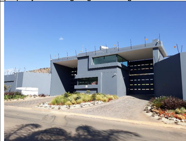
Photo 16: The securely guarded entrance to the site.
