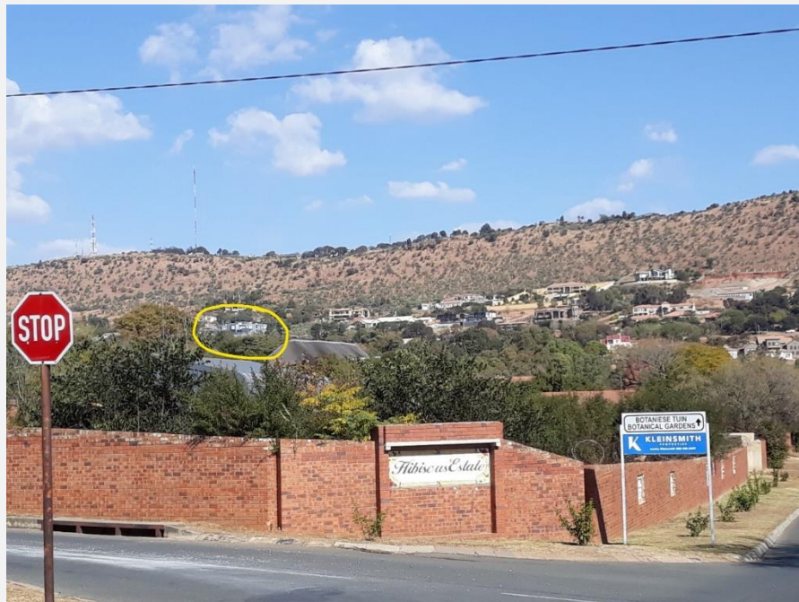
Figure 1: View looking back towards the property
