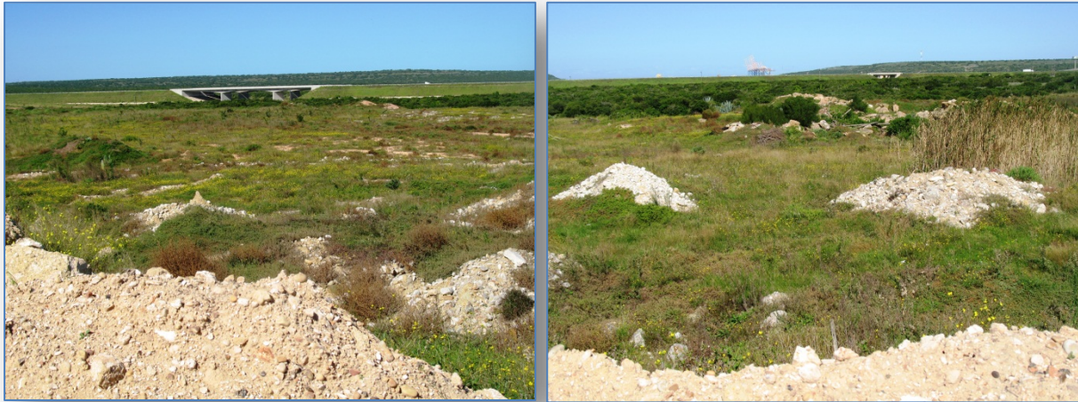
Figure 2.12: Proposed location of Manganese stockyard in relation to N2 bridge with associated Coega River flowing underneath (at left – looking eastwards) and port in distance (at right – looking southwards)
