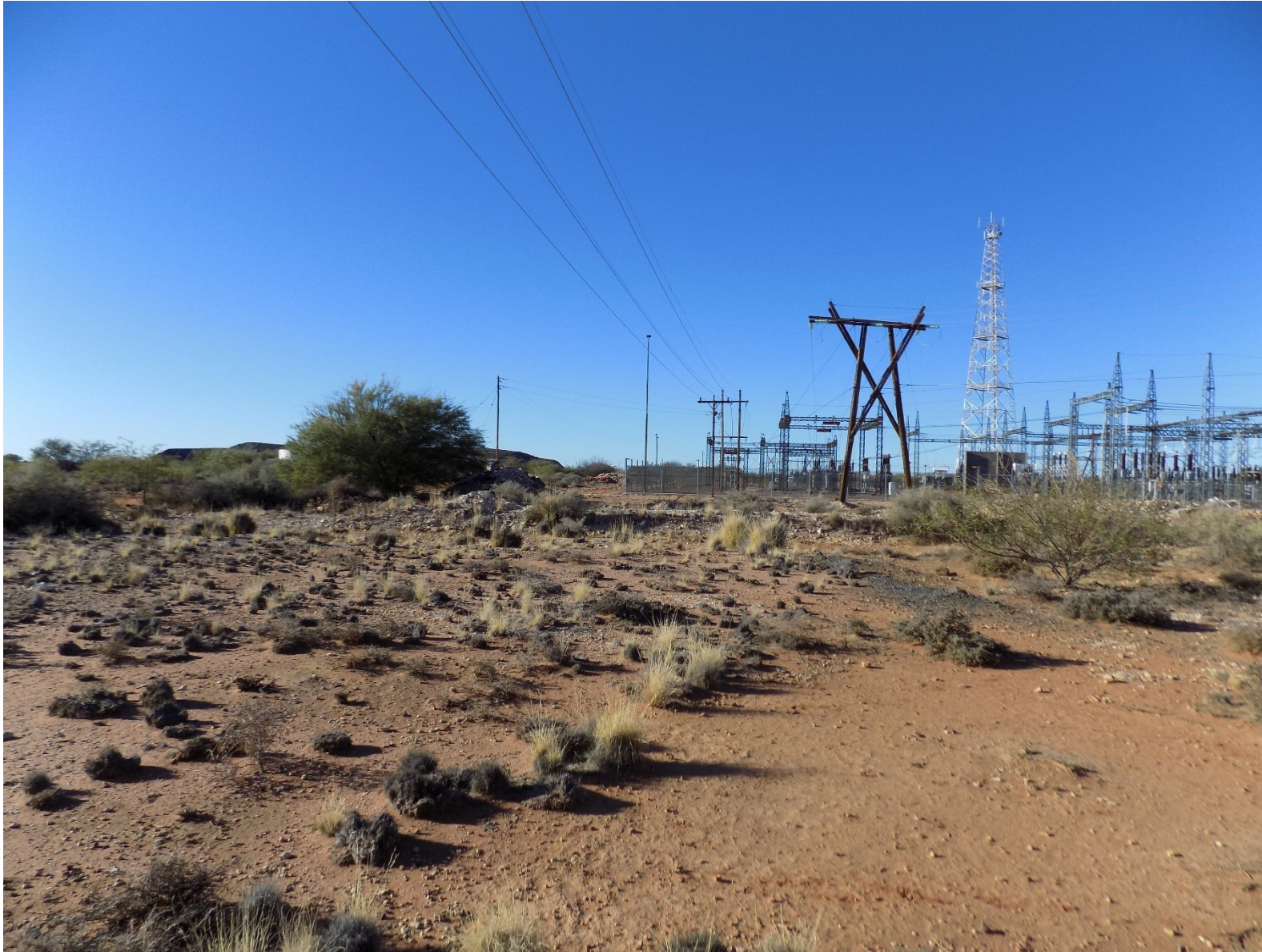
Figure 7 South west of the study area and proposed start location of the realigned 11kV and 66kV powerline (29°57'34.84"S; 22°17'56.80"E)
