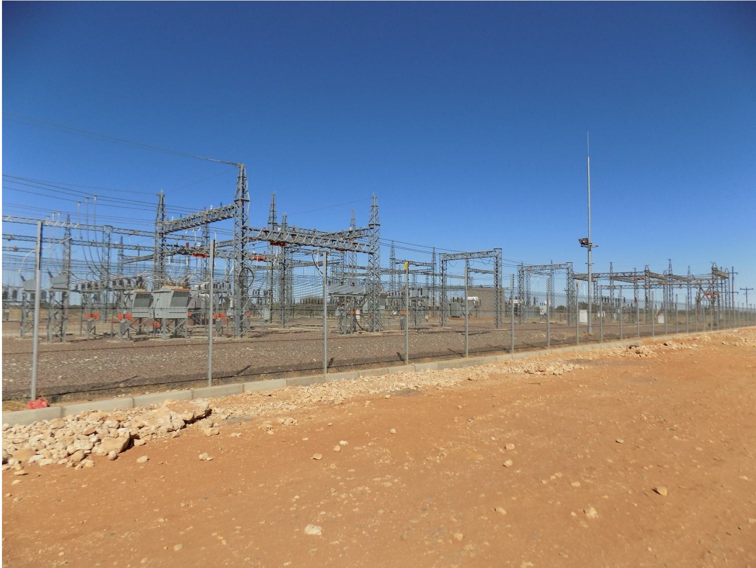
Figure 4 Cuprum substation viewed from west boundary of substation (29°57'31.96"S; 22°17'59.75"E)
