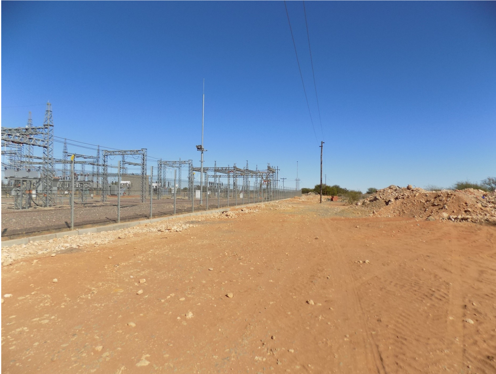
Figure 3 Cuprum substation viewed from west boundary of substation (29°57'30.78"S; 22°18'1.38"E)
