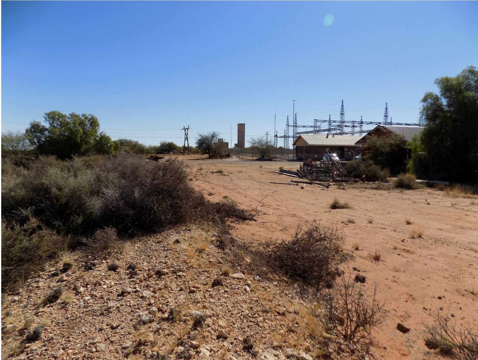
Figure 11 Location of the proposed BESS infrastructure viewed from south east of the study area ( 29°57'37.78"S; 22°18'1.51"E)
