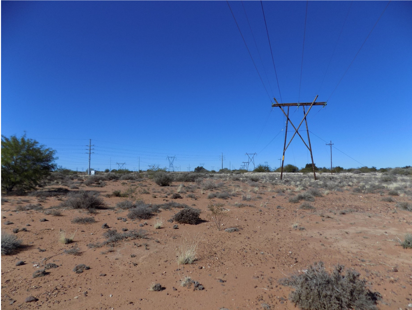
Figure 15 Location of the proposed 11kV and 66kV powerline realignment viewed from south of the study site (29°57'40.22"S; 22°18'0.75"E)
