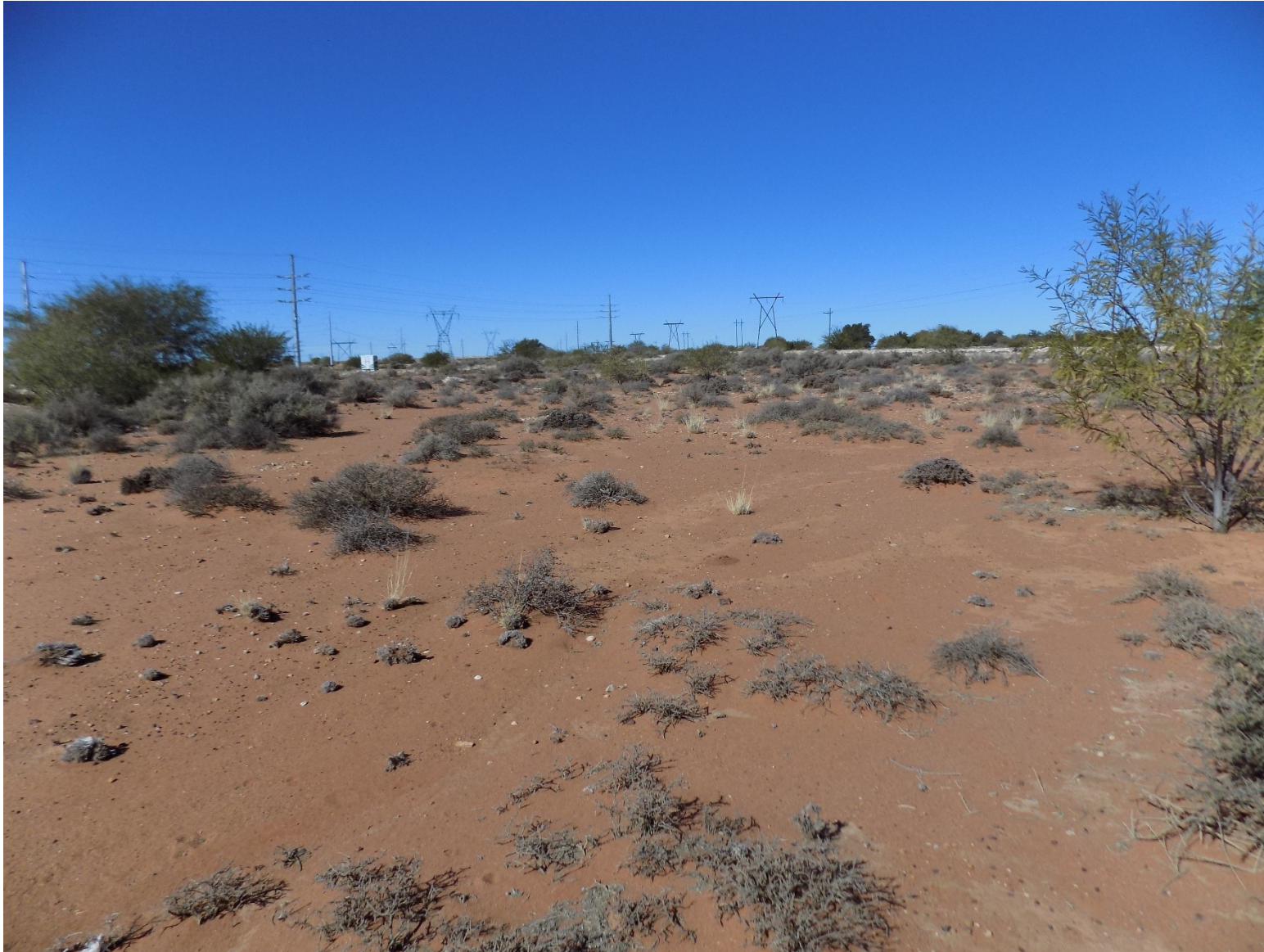
Figure 14 Location of the proposed 11kV and 66kV powerline realignment viewed from south of the study site (29°57'38.22"S; 22°17'57.53"E)
