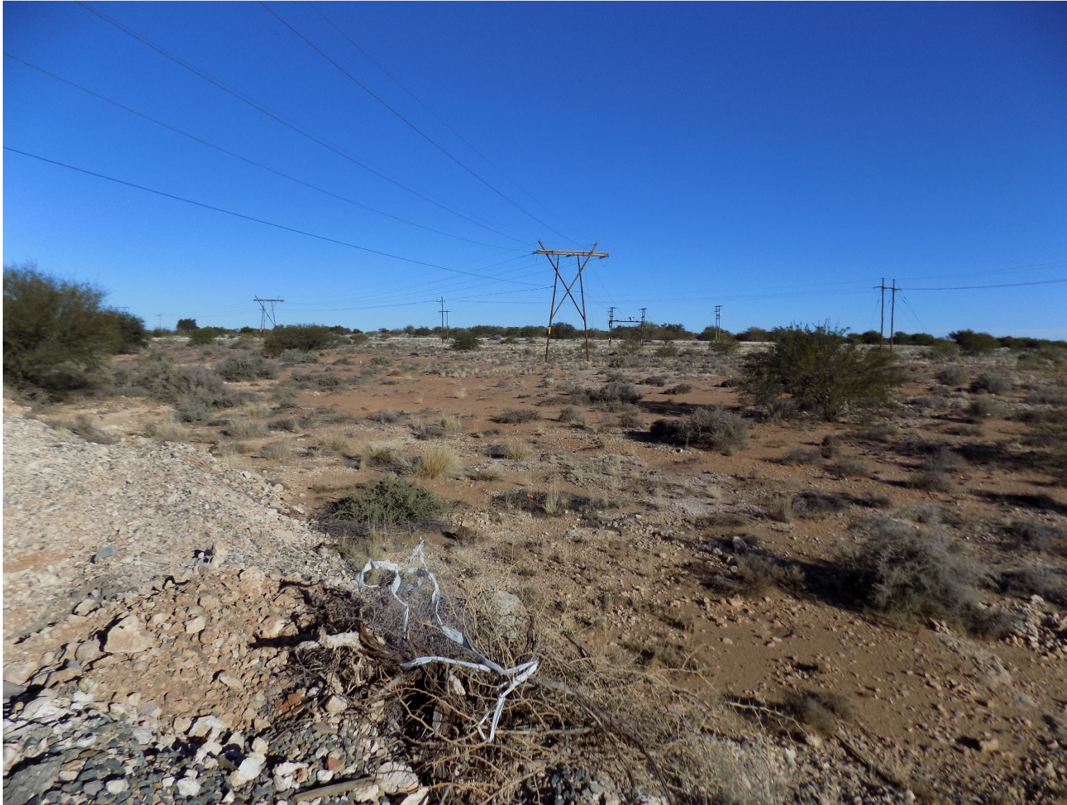
Figure 13 Location of the proposed 11kV and 66kV powerline realignment viewed from south of the study site (29°57'35.13"S; 22°17'57.68"E)
