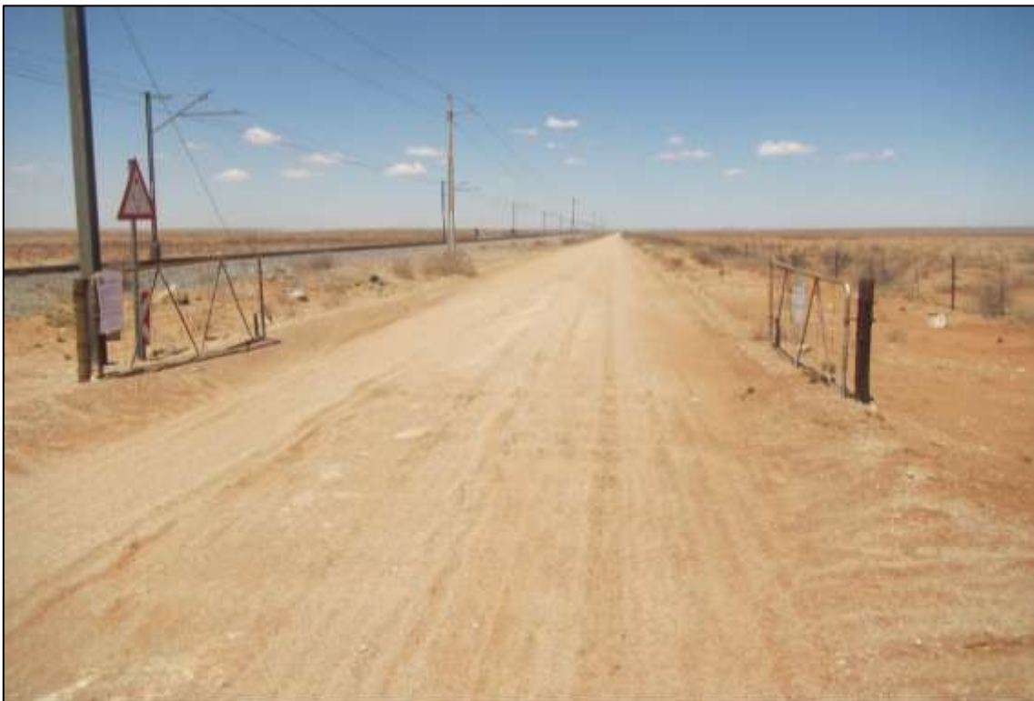
Figure 5: View towards the southwest along the existing Transnet service road (Option A) from the point at which access would be provided to the PV sites. PV1 lies to the right, PV2-6 lie to the left.
