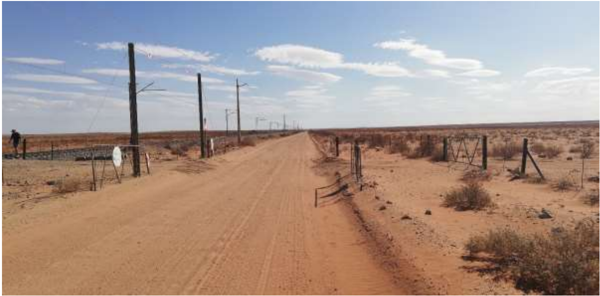
Figure 18: Existing Transnet Service Road
