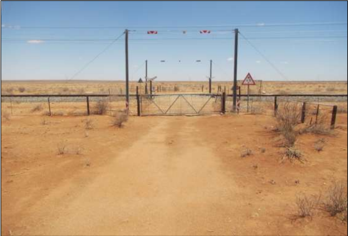
Figure 6: View towards the north across the existing level crossing where all access road options would cross the Transnet railway line. The Transnet service road is on the north side of the railway line.
