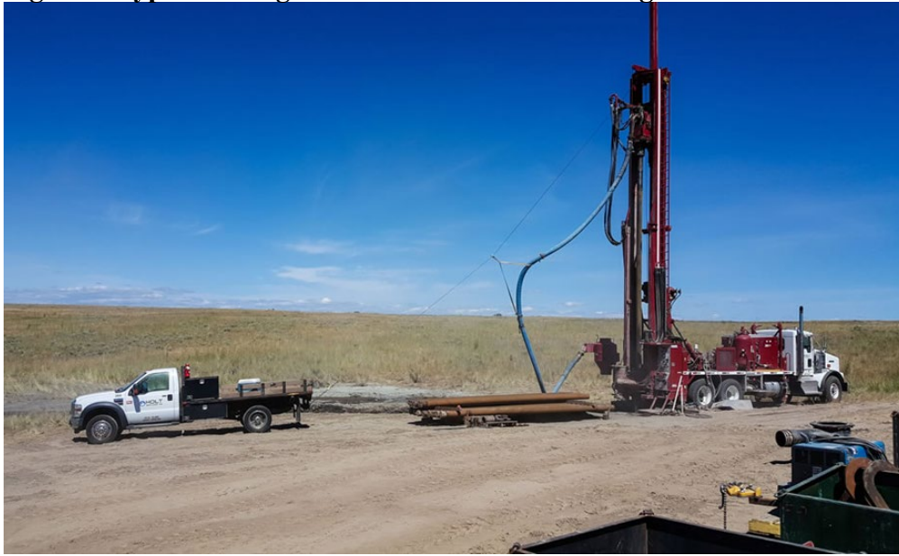
Figure 4 Typical configuration of a diamond drill rig
