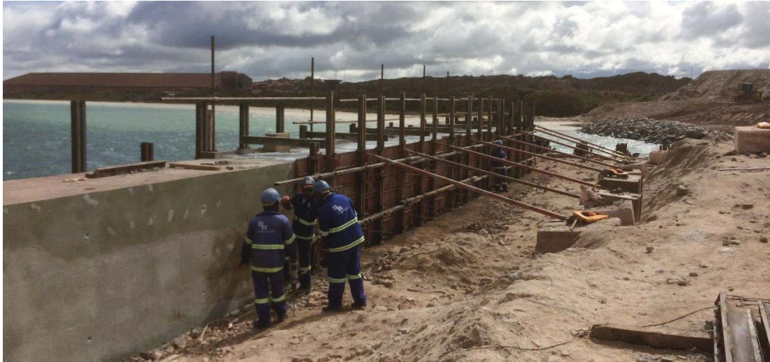
Figure 9-3: Concrete capping beam – South Africa, Saldanha Bay, General Maintenance Quay 2015
