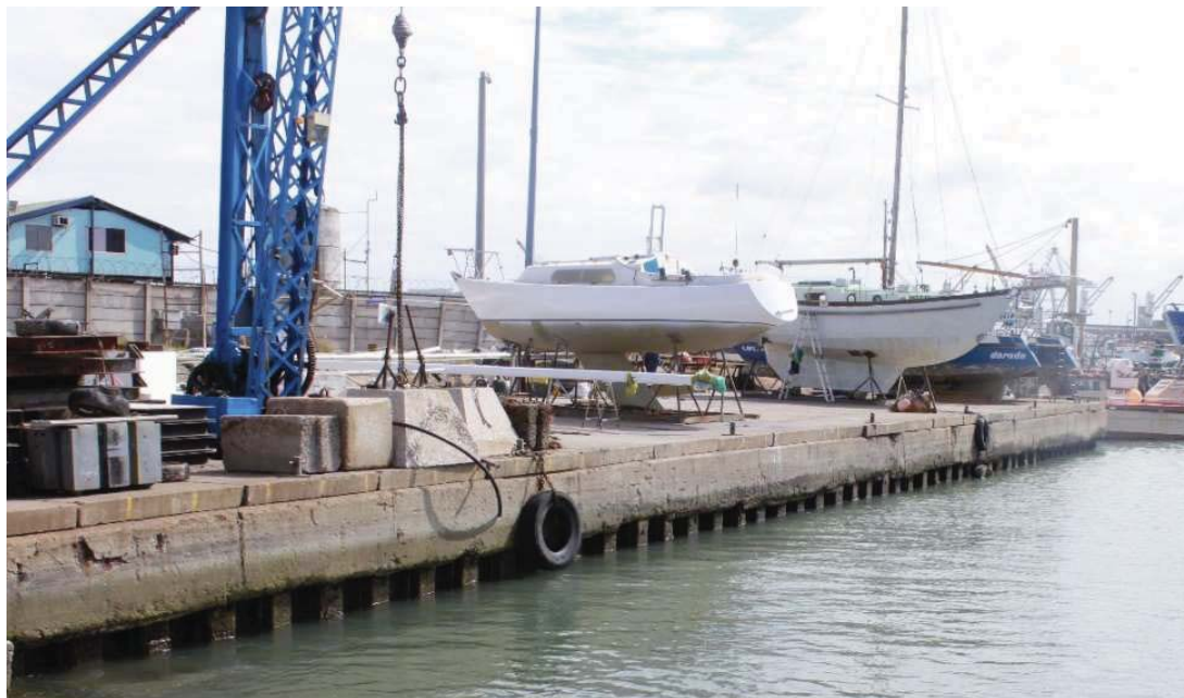
Figure 4-3: Southern side of Old Tug Jetty Sheetpile
