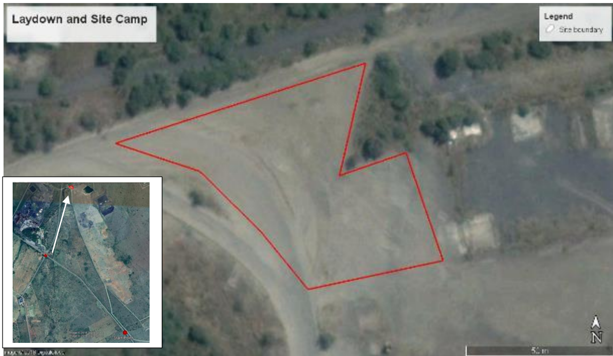
Figure 5.2: Aerial image of the Boshhoek laydown area and site camp (Source: GoogleEarth)
