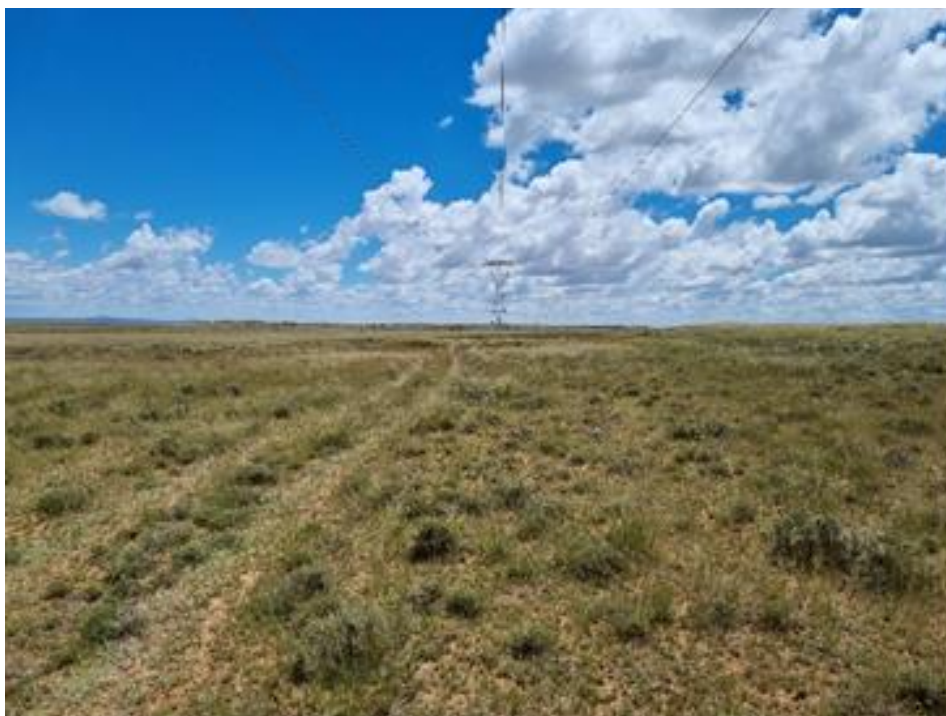
Photo 3. Existing 132kV ESKOM distribution line.
