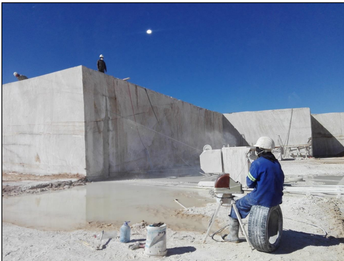
Photograph 2: Diamond-impregnated wire saw in action at Yellow Quarry 1.
