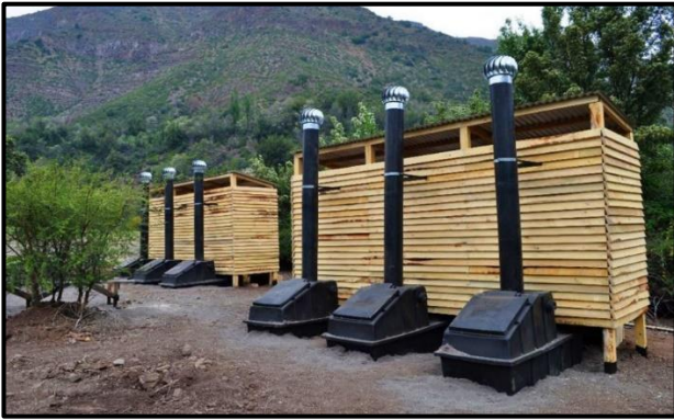
Diagram 8a: Example of a dry enviro loo system
