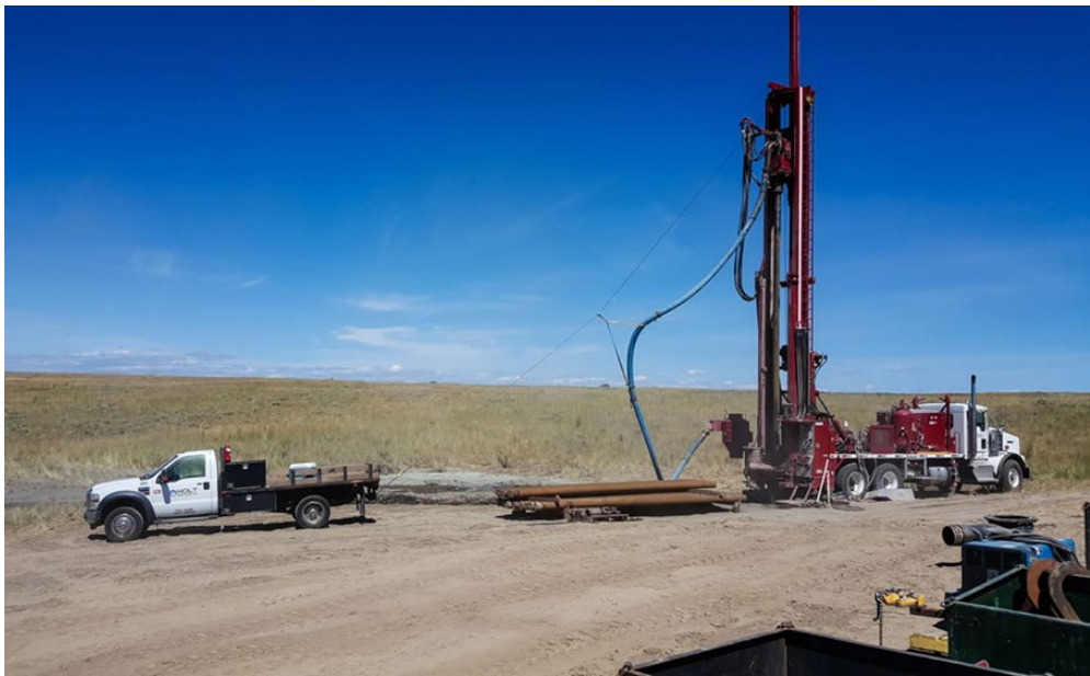
Figure 4 Typical configuration of a diamond drill rig
