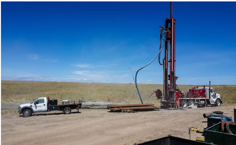
Figure 4 Typical configuration of a diamond drill rig
