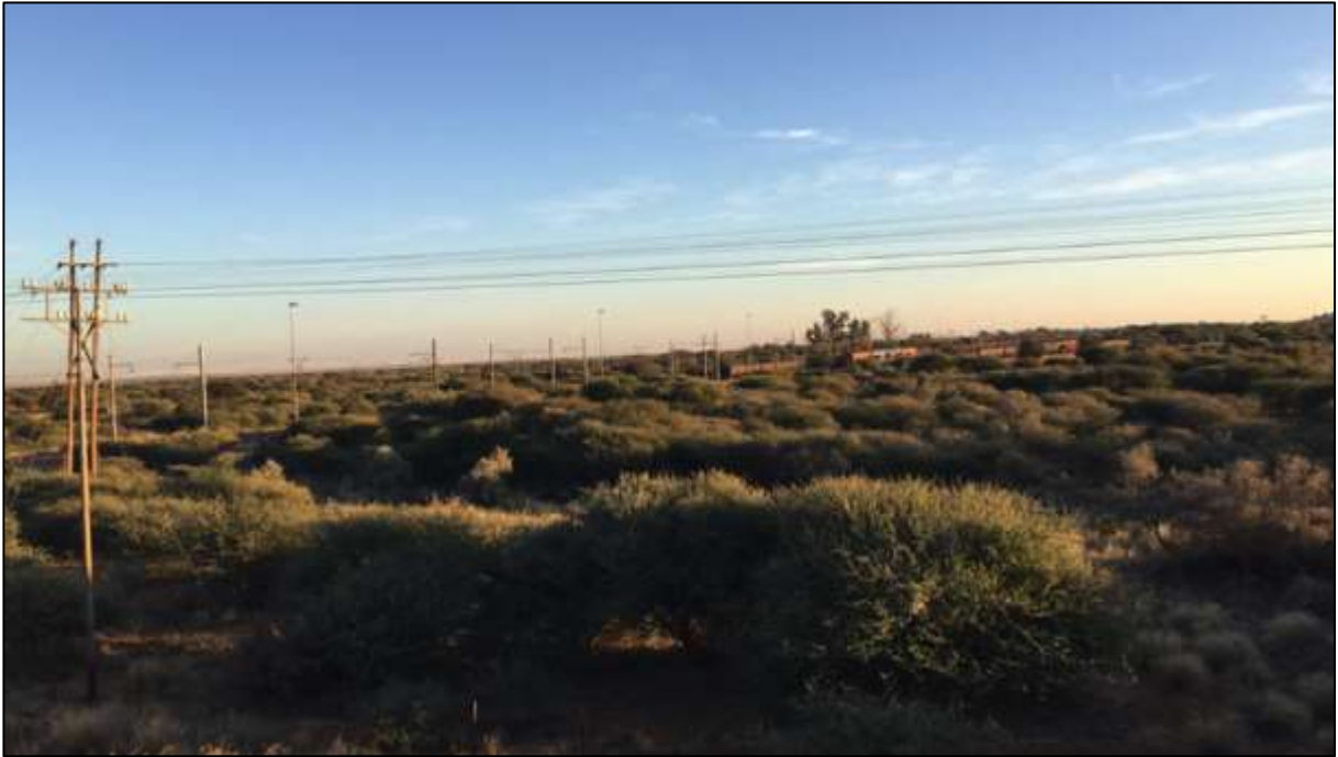
Figure 6: View north from Photo 5 of the existing power line and railway line infrastructure along which the proposed power line would be routed.
