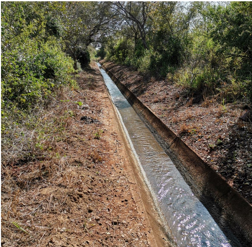
Figure 4: Canal located at 25° 29'50.81"S 31° 31'24.92"E
