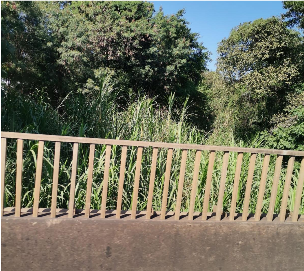
Figure 7: Bridge crossing the Buffelspruit
