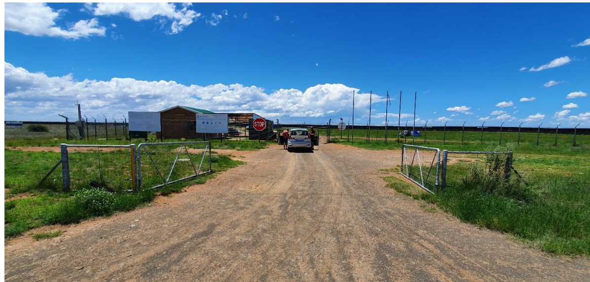
Figure 3: Access control to Pulida PV Facility
