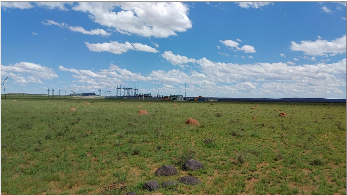
Figure 8: View of Pulida PV and substation
