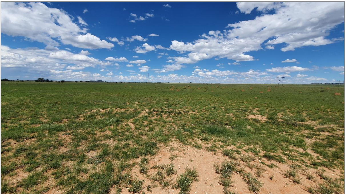
Figure 9: View of facing towards existing transmission lines leading from substation
