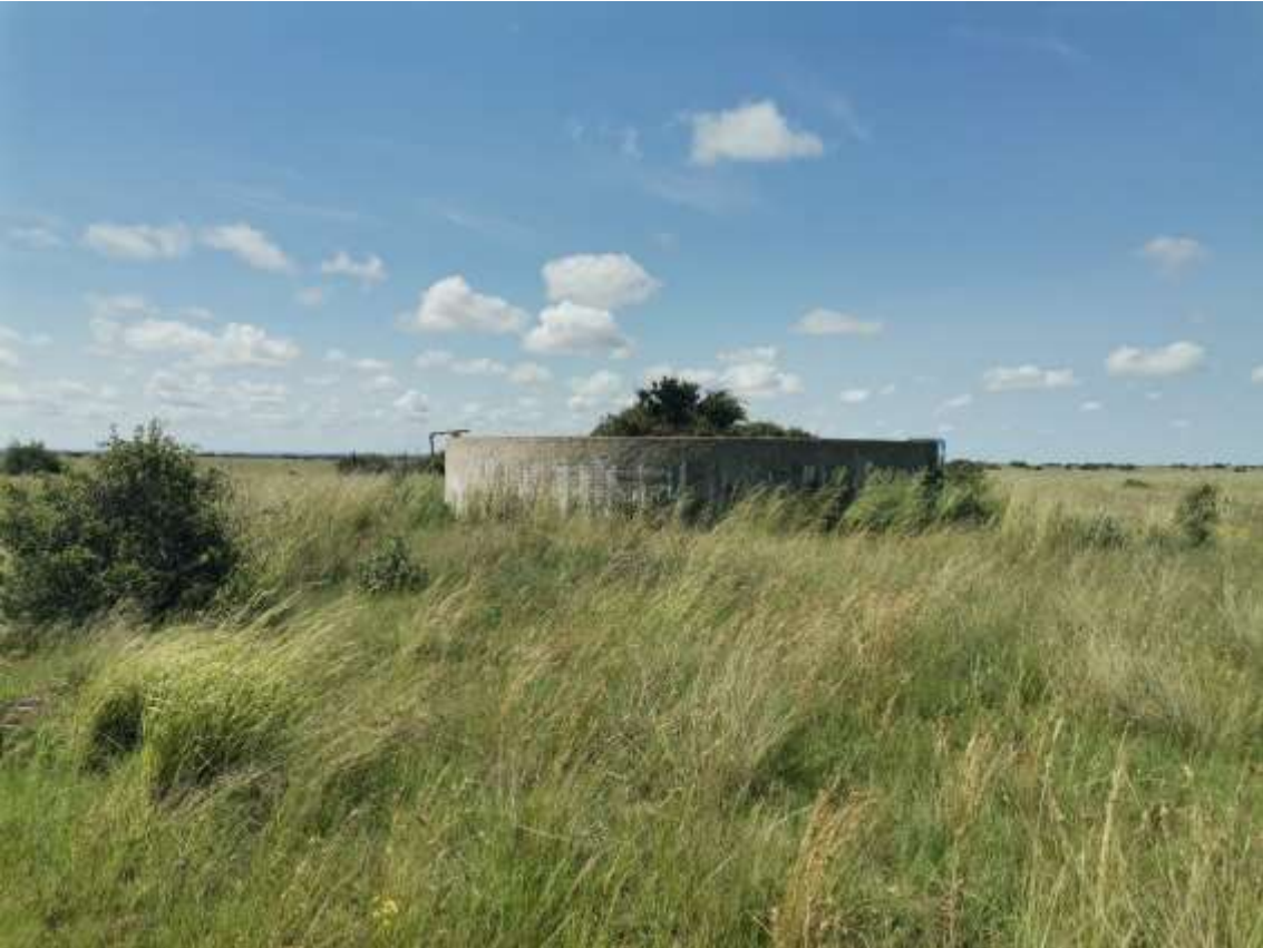
Figure 5: Existing Water Reservoir on site
