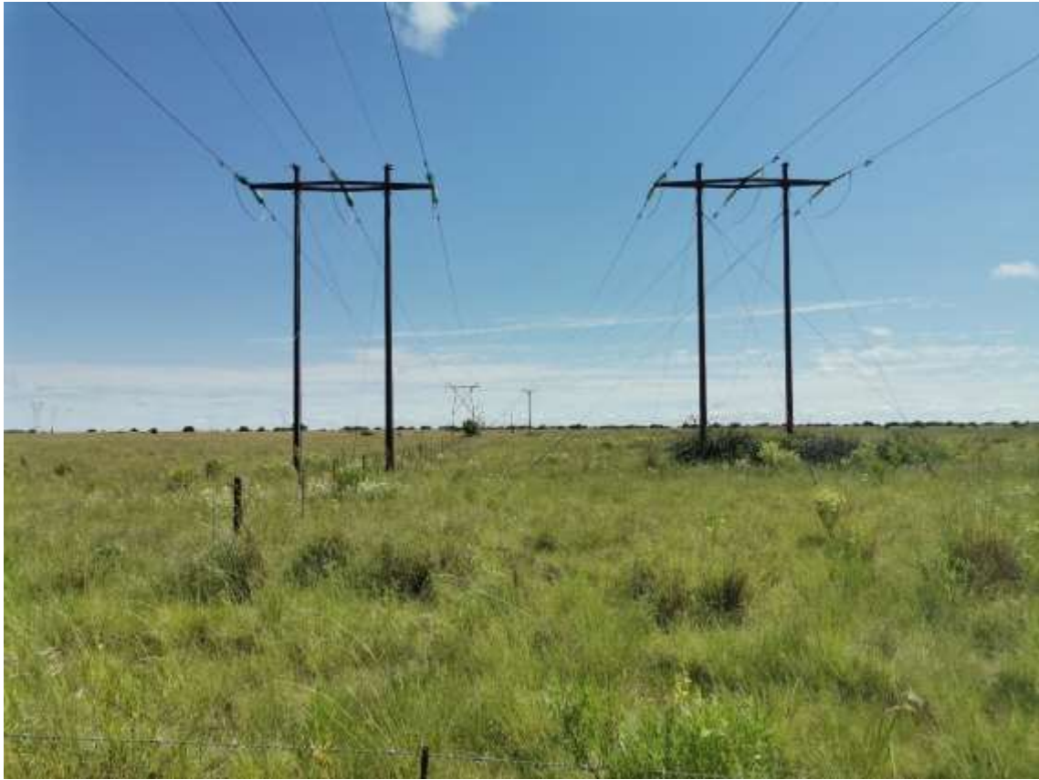
Figure 12: Existing powerlines traversing the property
