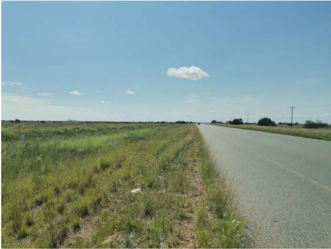
Figure 10: R503 running adjacent to the site
