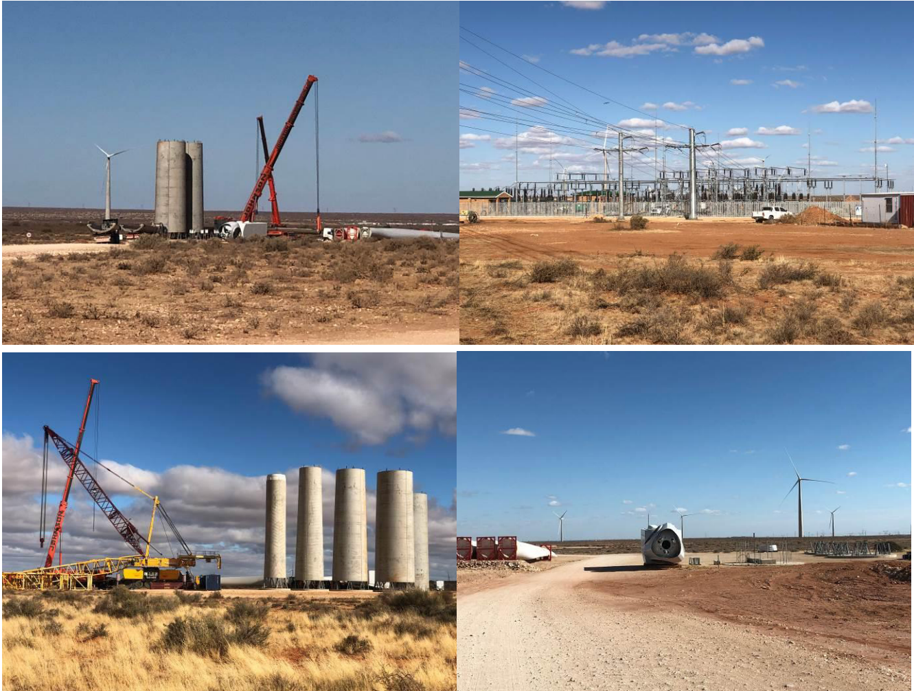
Figure 2-4: Photographs depicting the construction phase of a wind farm similar to De Rust North WEF.
