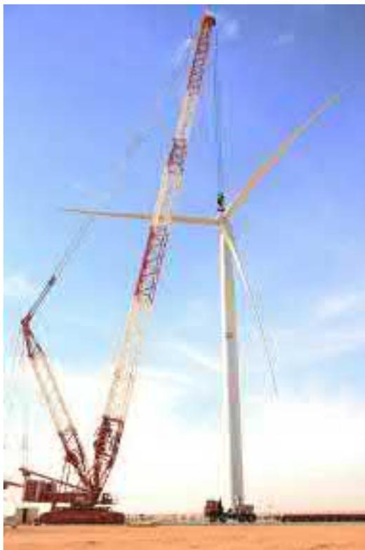
*Figure 4-5: Crawler Crane used to assemble turbine (Liebherr, 2017)*
