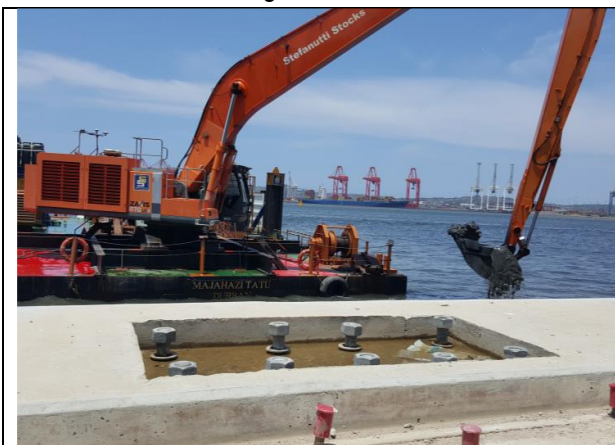
1. Dredge to required level
