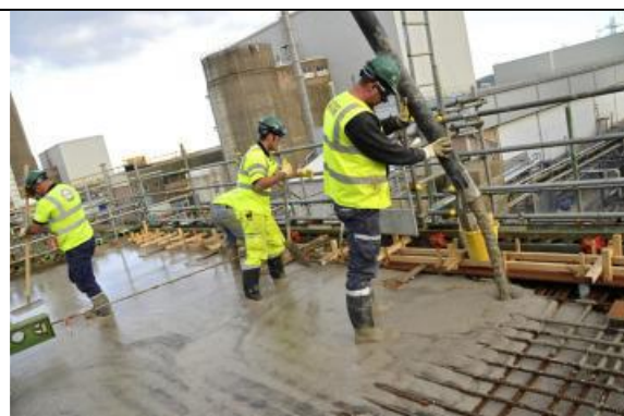
5. Install civil services & place stitching concrete
