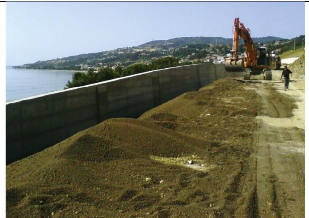
4. Backfill & install civil services
