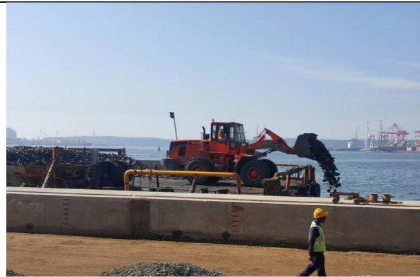
3. Place scour rock
