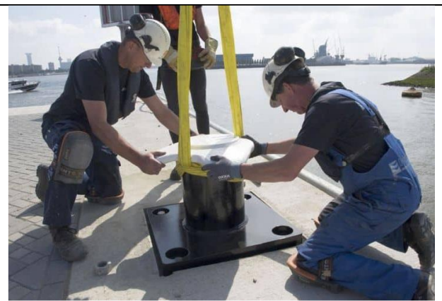
6. Pave & install quay furniture
