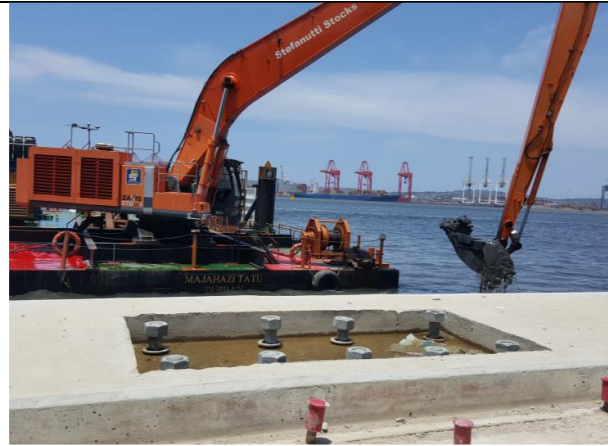
1. Dredge to required level
