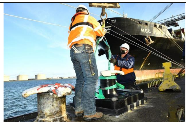
6. Install quay furniture
