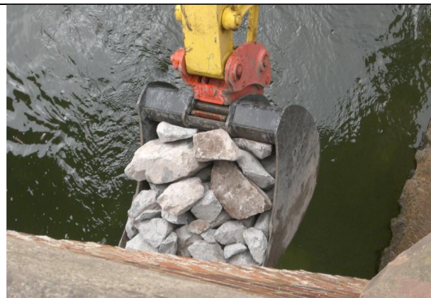
3. Place scour rock
