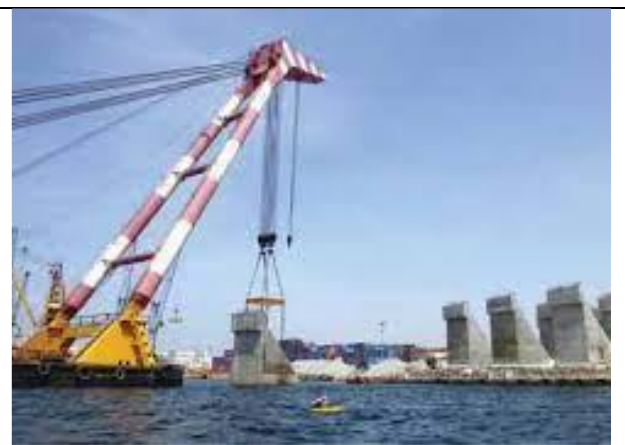
2. Place counterfort units & block work
