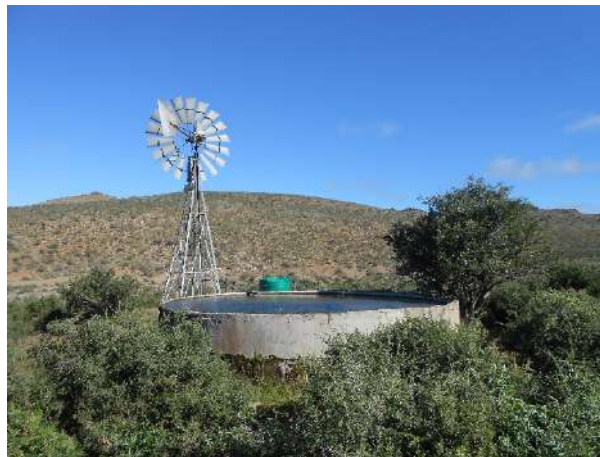
W29: Working wind pump and reservoir with water
