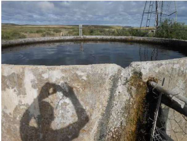
W1: Working wind pump, reservoir with water, and trough with water
