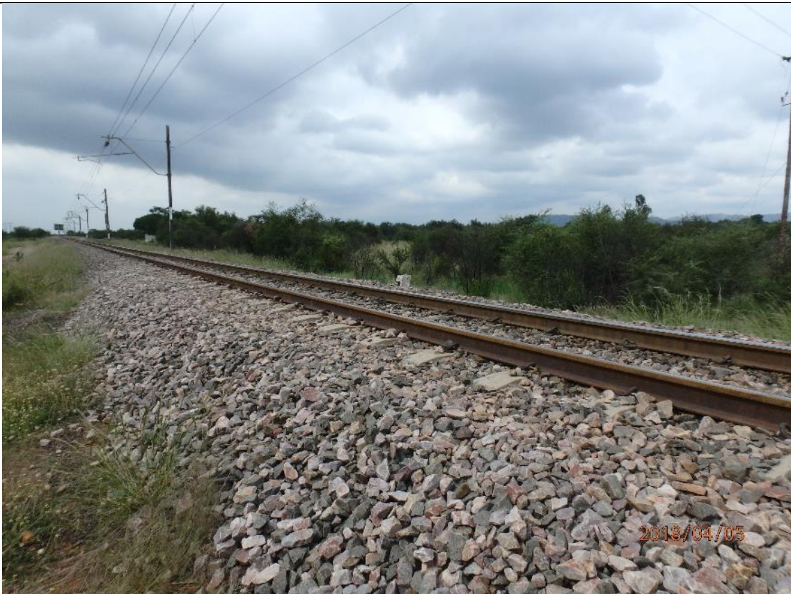
General view of the existing railway line.
