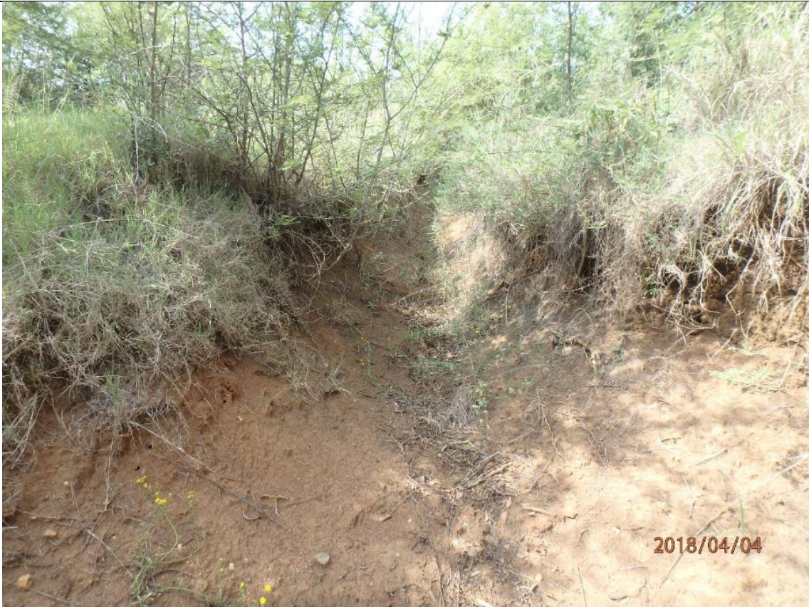
Drainage line filled with terrestrial vegetation immediately adjacent the railroad at culvert No. 2 (on Figure 4.10). GPS coordinates: 25°30'37.41"S, 27° 7'5.99"E.
