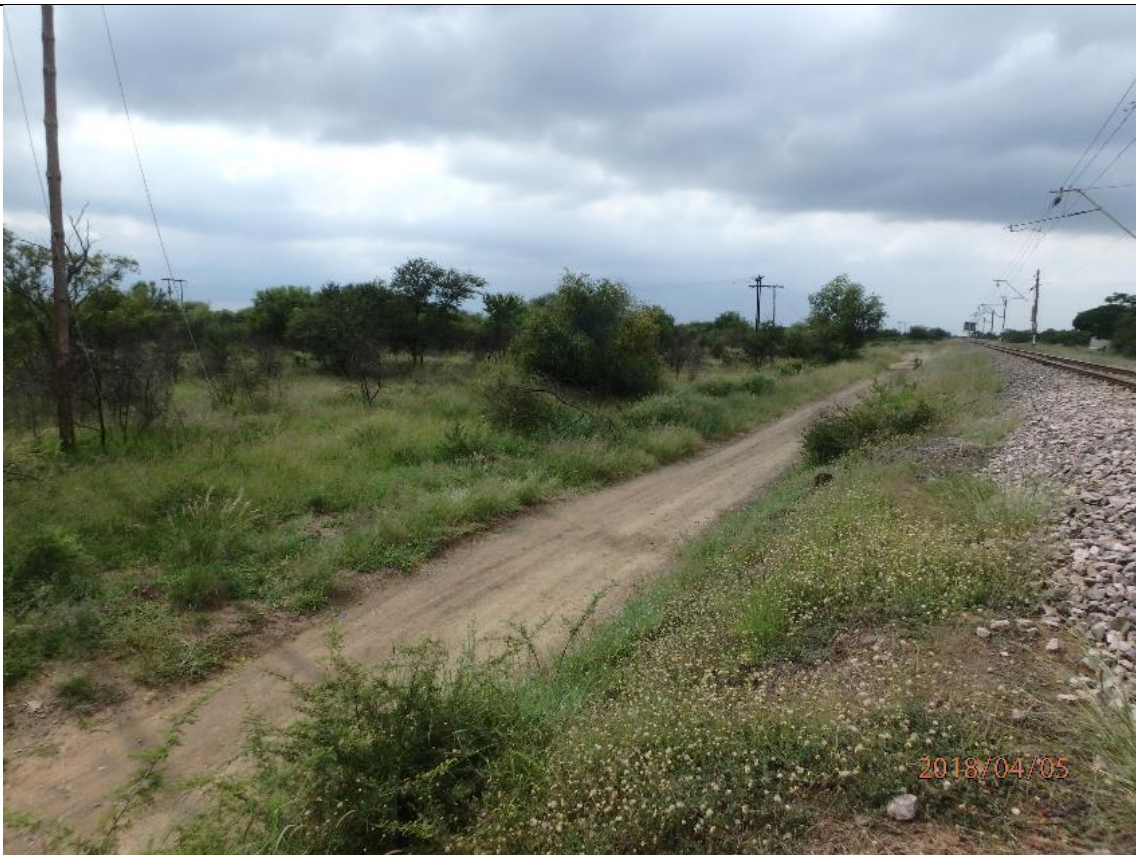
General view of the railway on the northern facing side, with access road present.
