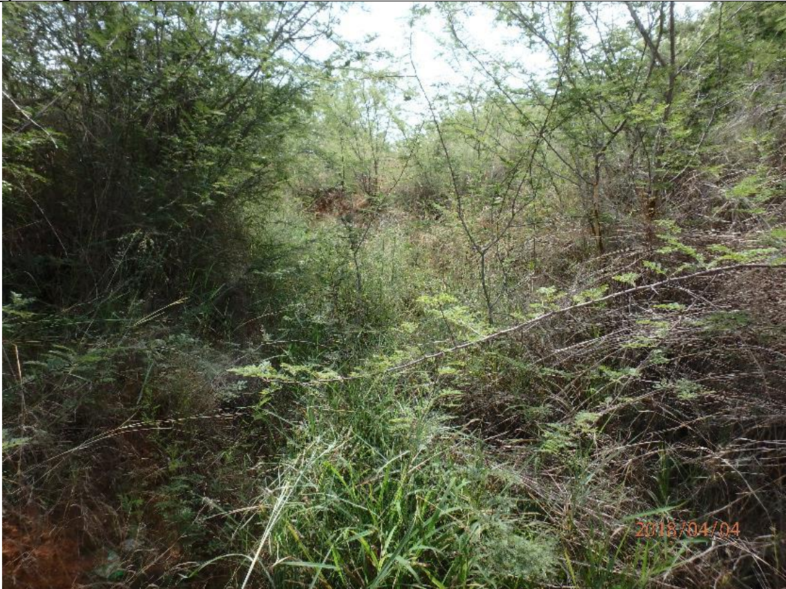
Drainage line filled with terrestrial vegetation immediately adjacent the railroad at culvert No. 3 (on Figure 4.10). GPS coordinates: 25°30'16.03"S, 27° 6'46.17"E.
