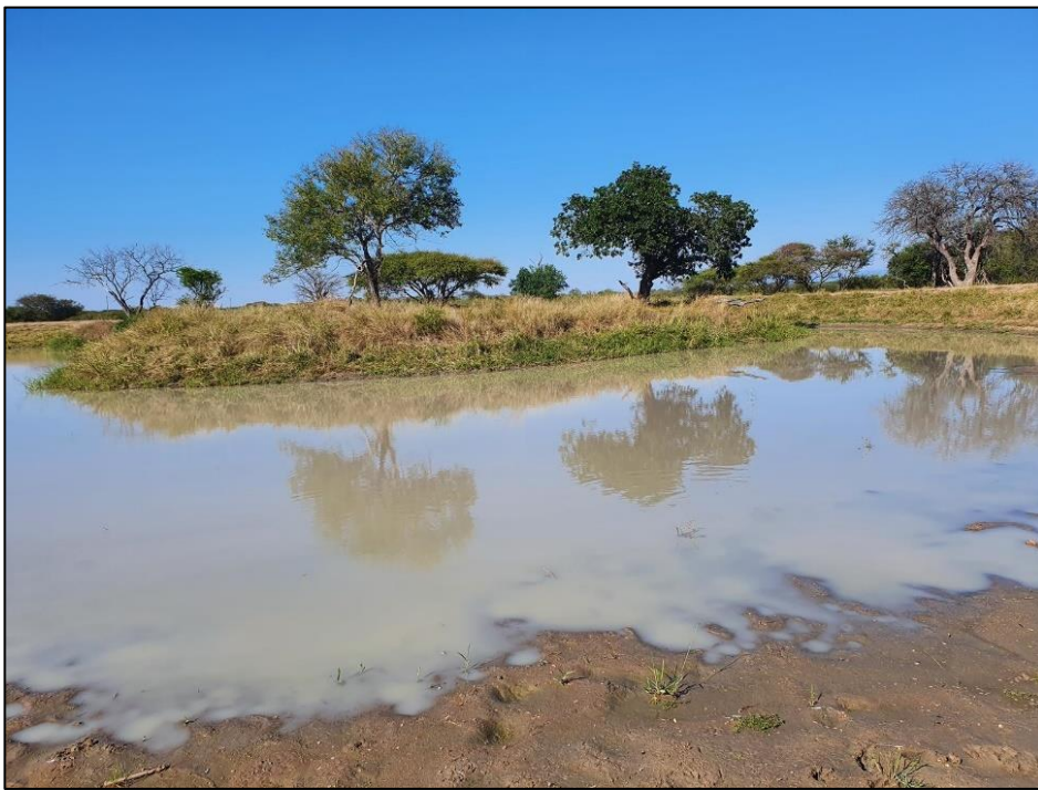
Earth Dam at Schoongezicht 66 KU. [2021-07-21].
