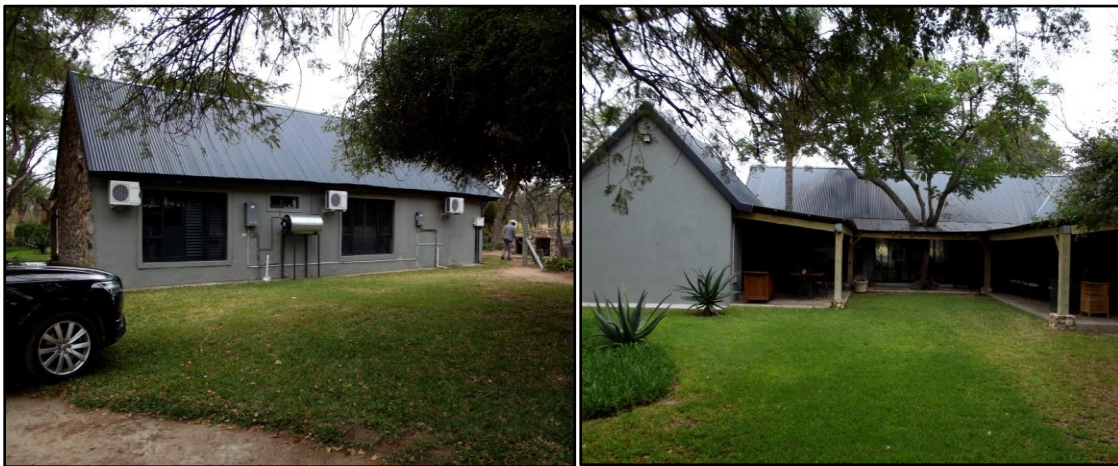
Fig. 4. Site S3. Photos taken towards the north-west and north.
