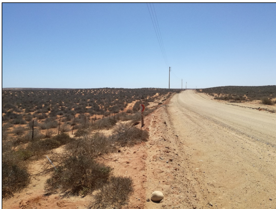
Figure 13: View of 66 kV power lines along the Komaggas-Kleinsee link road
