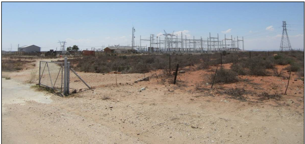
Photograph 3.7: Eskom's Gromis Main Transmission Substation located 11 km to the north-east of Kleinsee
