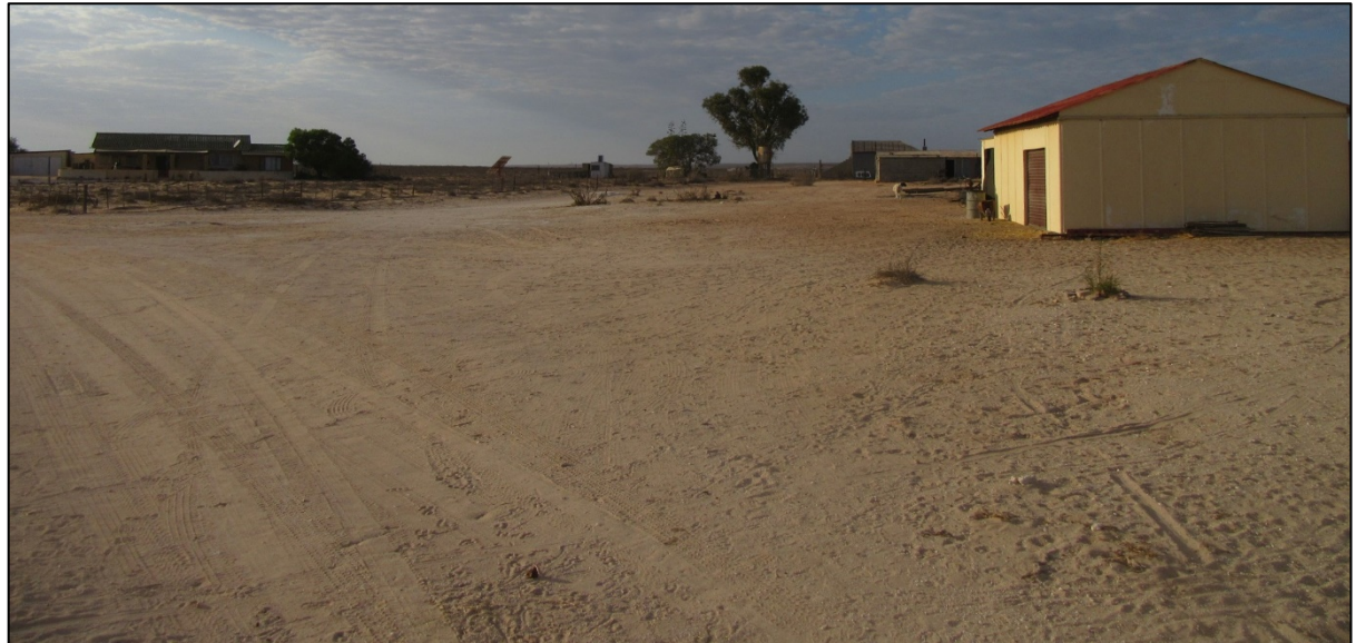
Photograph 3.13: Rooivlei (D Engelbrecht) farmstead and outbuildings. The Namas WEF has been approved on this portion of Rooivlei Farm.
