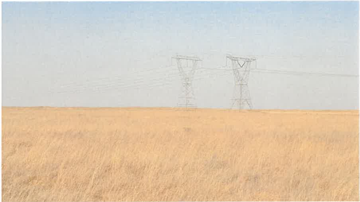
Kinderdam substation site looking east:
