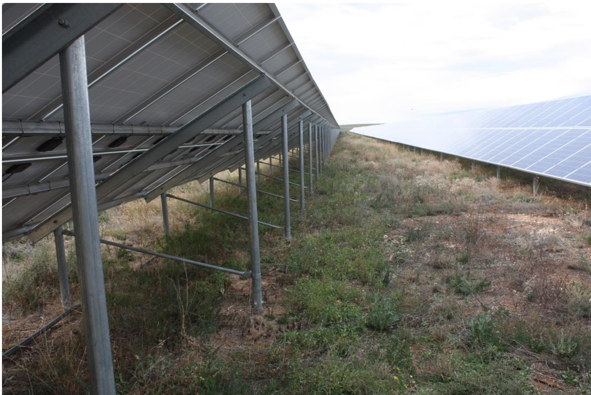
Figure 13: Image of solar arrays indicating the limited Influence that such structures generally have on the flow of surface waters within a solar facility.
