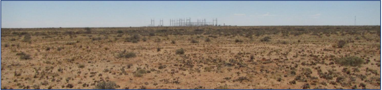
Figure 7: View towards the east along the northern part of the powerline corridor with the Nieuwehoop Substation visible in the background.
