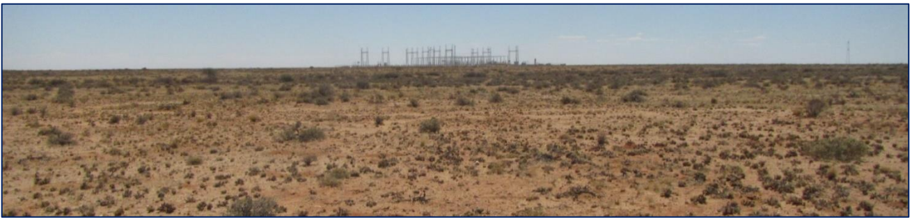
Figure 7: View towards the east along the northern part of the powerline corridor with the Nieuwehoop Substation visible in the background.
