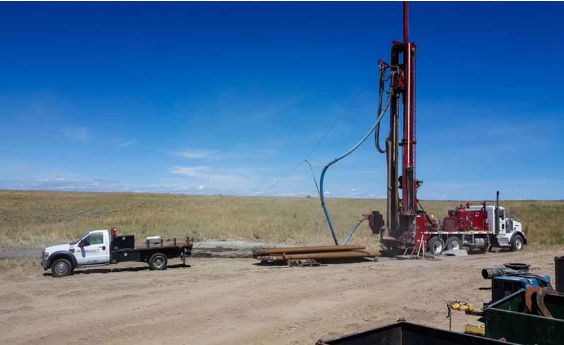
Figure 4 Typical configuration of a diamond drill rig
