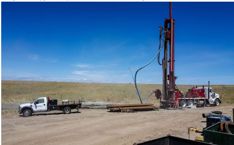
Figure 4 Typical configuration of a diamond drill rig
